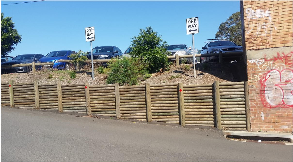
Photo 10: Timber retaining wall along the north eastern side of the property to be reconstructed.
